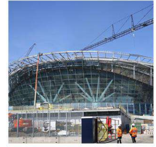
Sports Ground Construction
