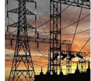
Substation & Transmission Line Works
